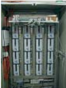
Figure 3/14 Passerelles EIB- BACnet (BUS-House)
