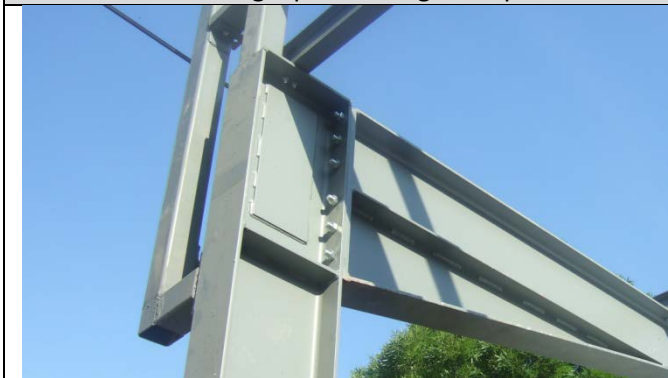
Assemblage traverse/poteau
