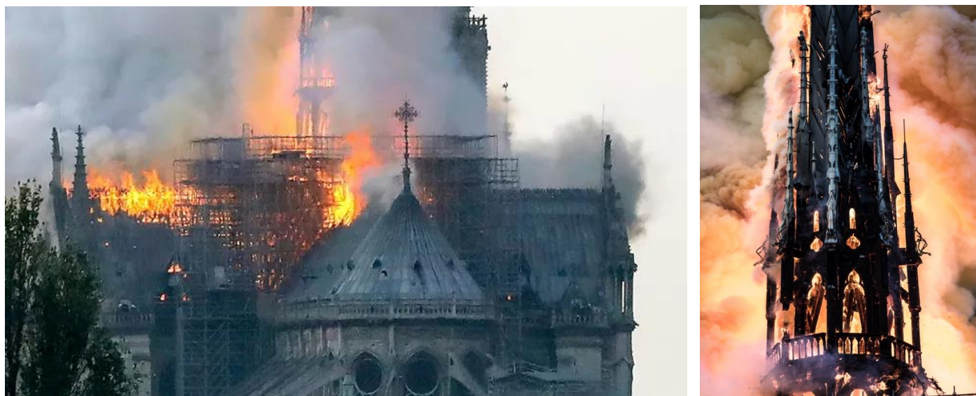
Figure 5 : Charpente et flèche en flamme, sources [7] [8]
