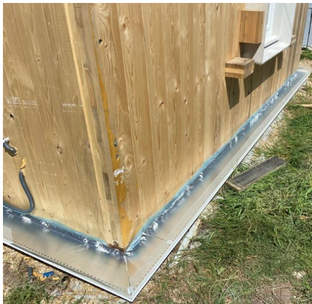
Figure 45 : Pose du rail supportant l'isolant
